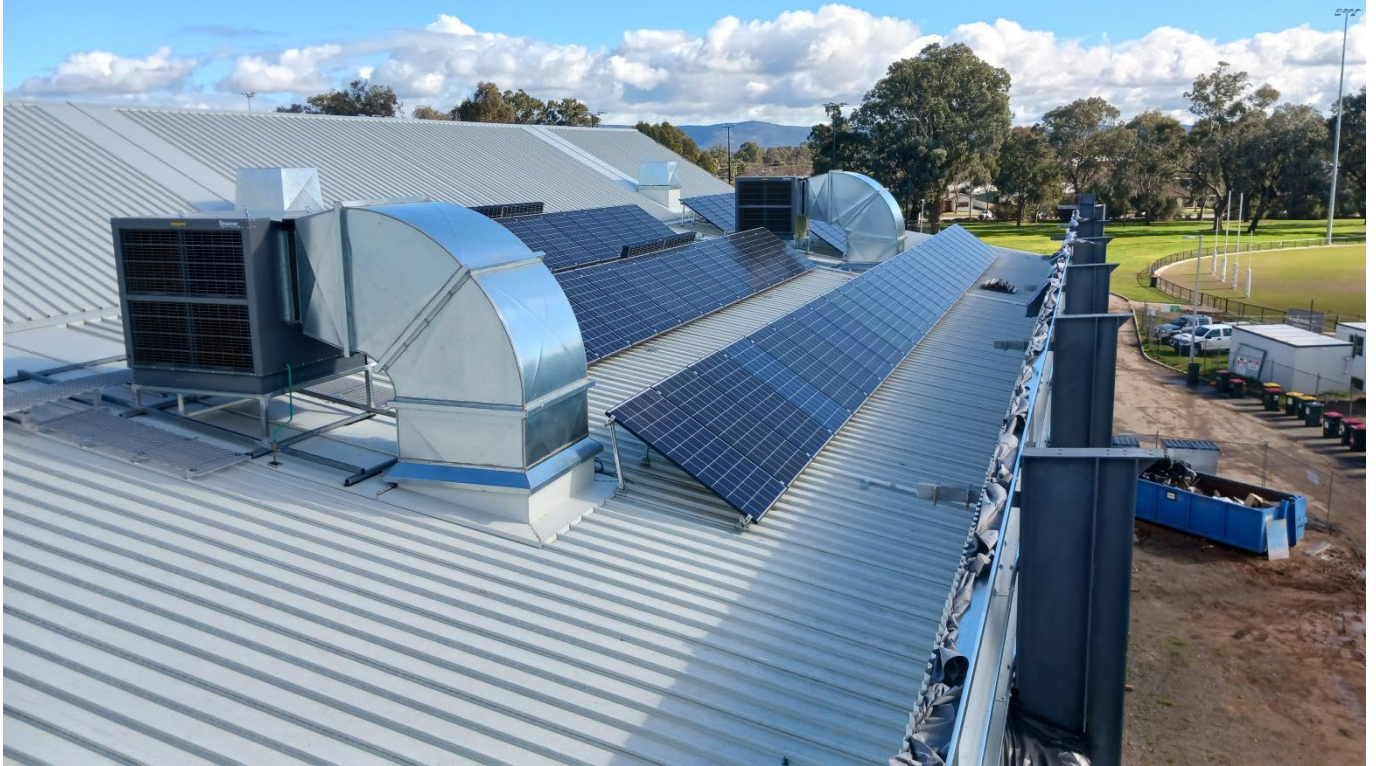
WSAC will have a total of 98 kW of solar panels feeding power into the facility.
