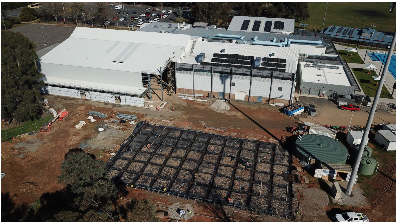
Show Court No 1 structure and Court No 5 footings prior to pouring of 243m 3 of concrete.
