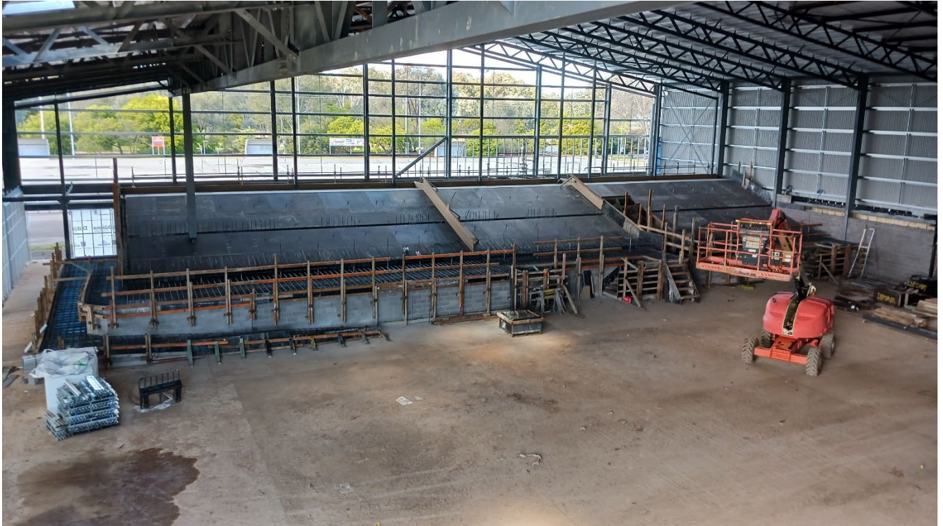
Show Court No 1. New East Grandstand formwork
