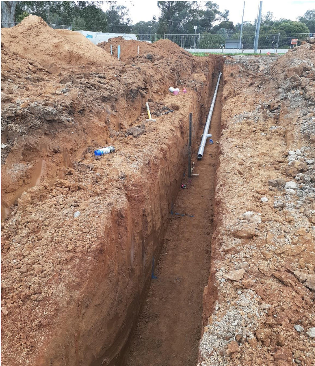
New sewer main installation (Oct 2022)
