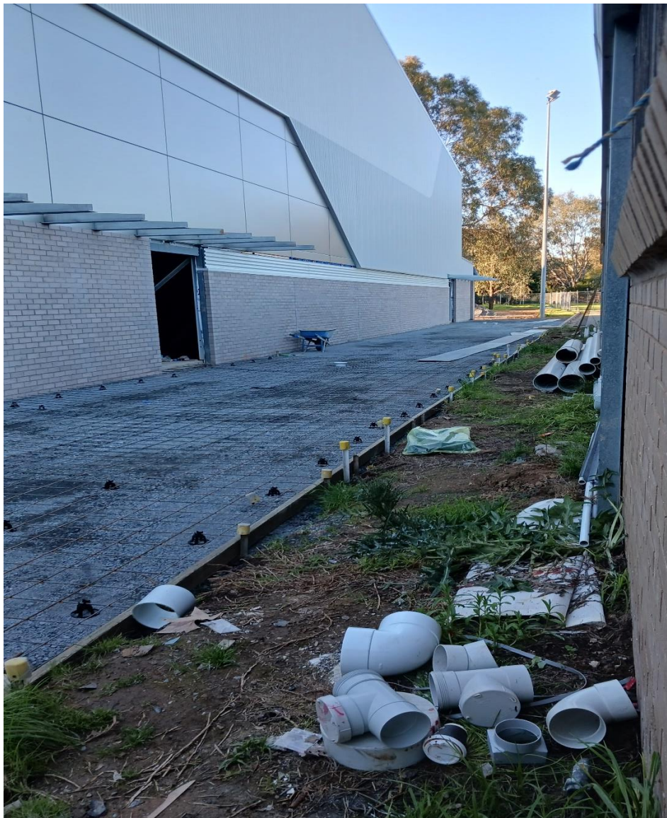
Concrete Pathway prepared for concrete (11 th September)
