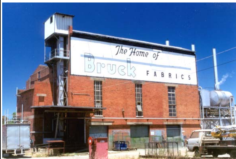
( 247-c19-09a.bmp ) The second Bruck boiler house, which generated steam for use within the textile mill.
