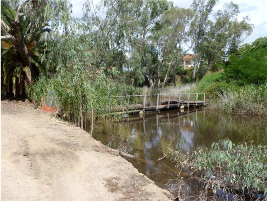
Photo of footbridge to be removed.
